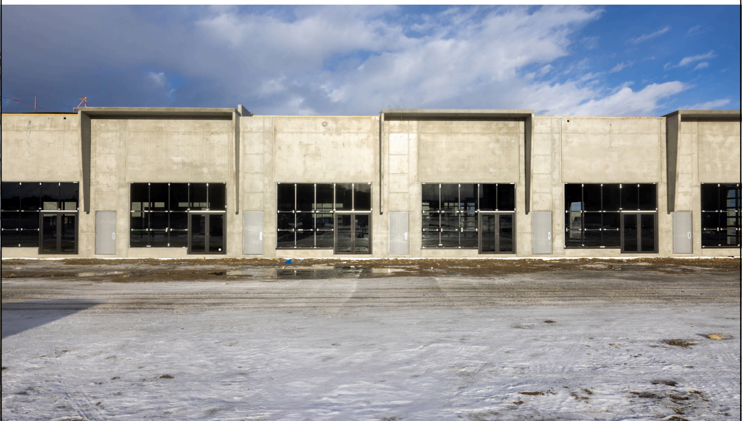
Construction images as of February 2025. The development is approximately 80% complete.
